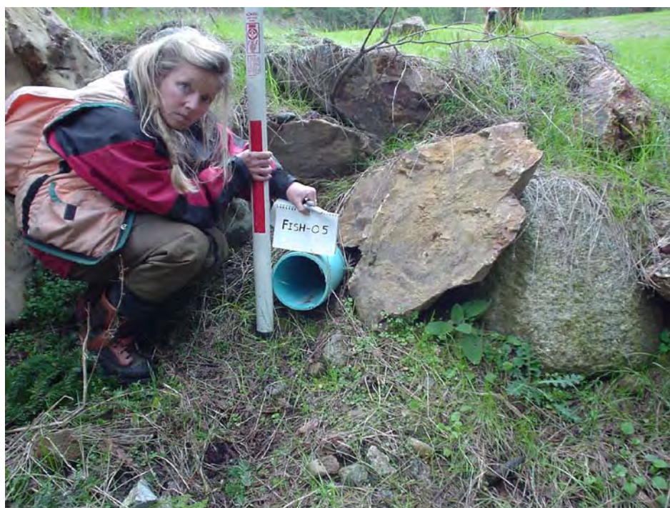
Photo Point N - Photo 30: Outlet of the Fish-05 pipe; a closed valve on this pipe prevents lake flow from entering Fishtrap Creek.
