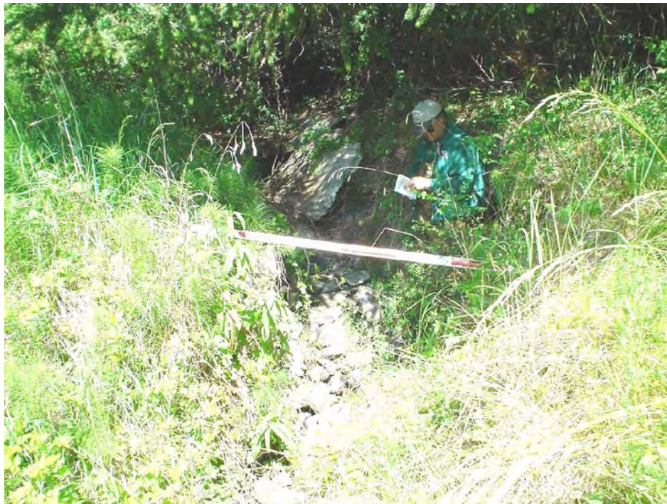
Photo Point B - Photo 3: Broken concrete spillway with 2 ft vertical drops between broken spillway slabs. The channel downstream of the spillway is completely rip rapped with a 20% gradient.
