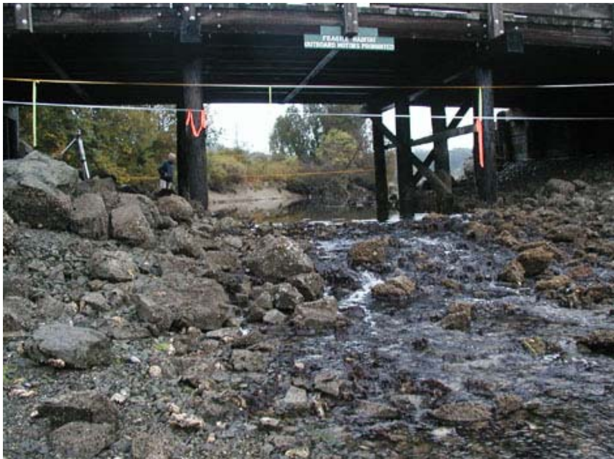
Figure 2. This photo is looking northward into Cayou Estuary to show the rock dam under the existing bridge. Notice the ponded water in the estuary.
